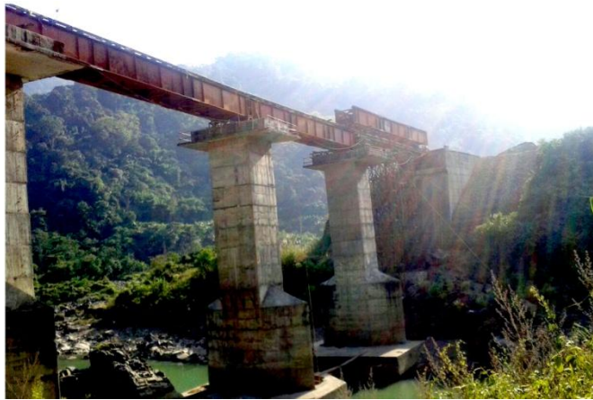
Bridge No. 4/13 of Lumding-Silchar GC section
